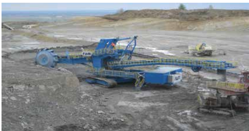
Figure 2, The “new” bucket wheel excavator.
