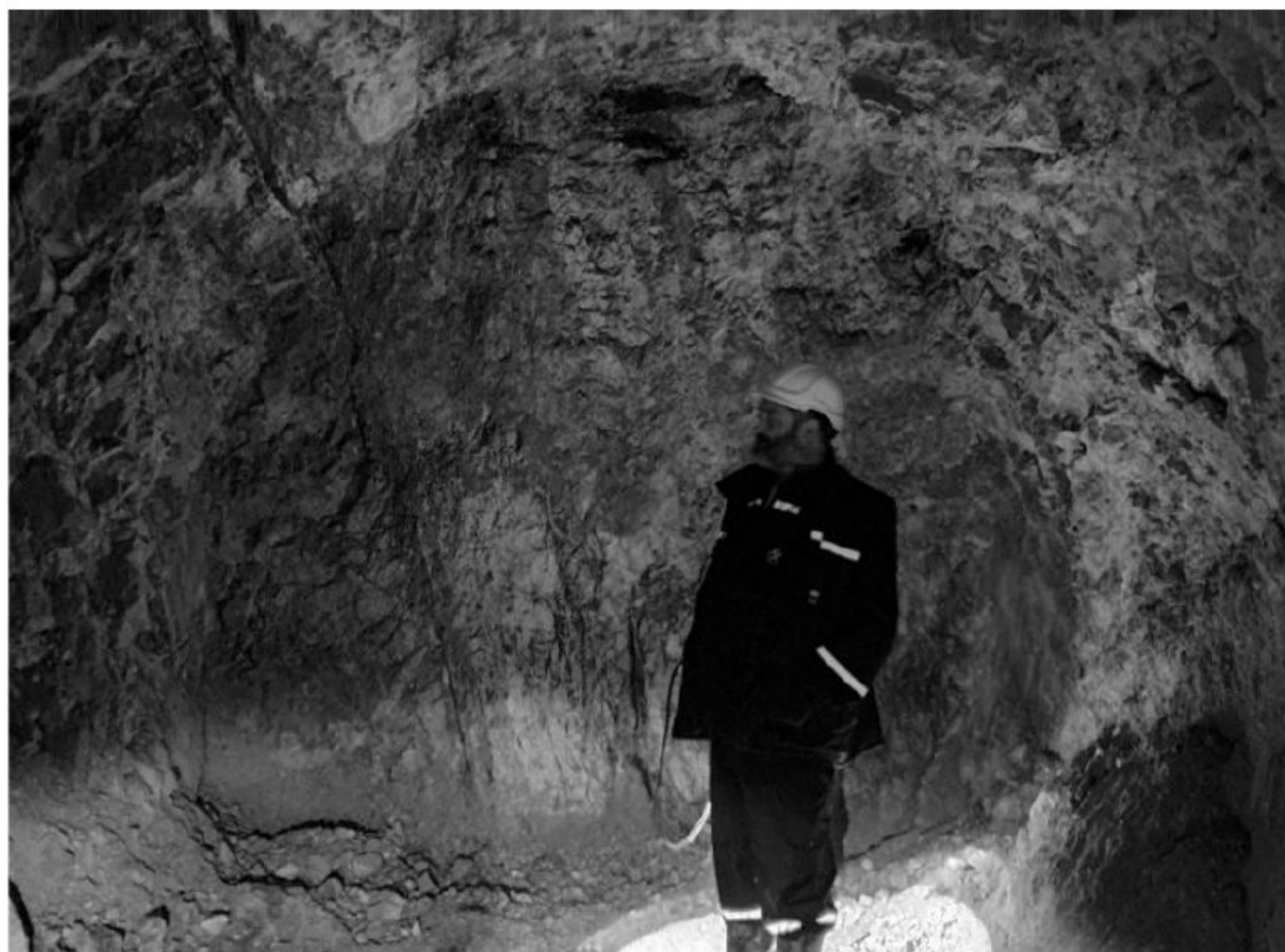
Figure 8 Drift excavated using cylindrical cut with circular initiation and contour blast
