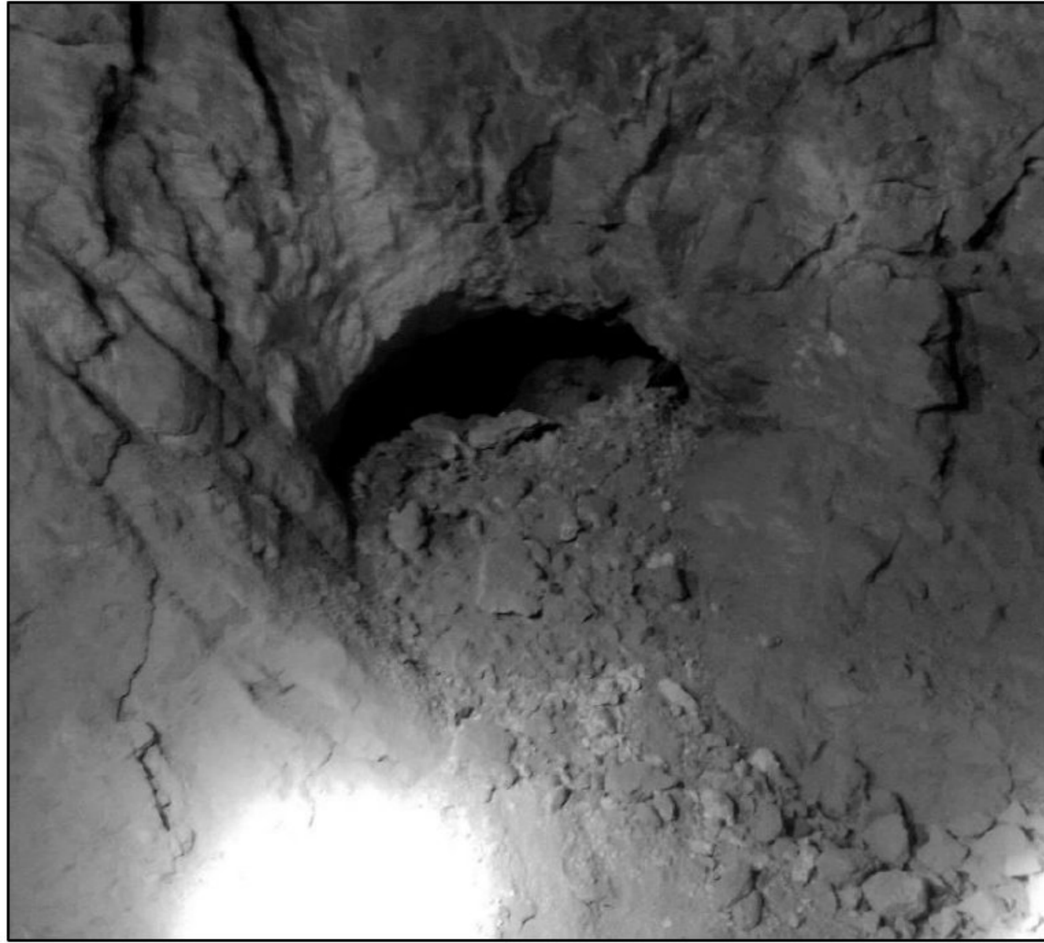
Figure 7 Results obtained after blasting
