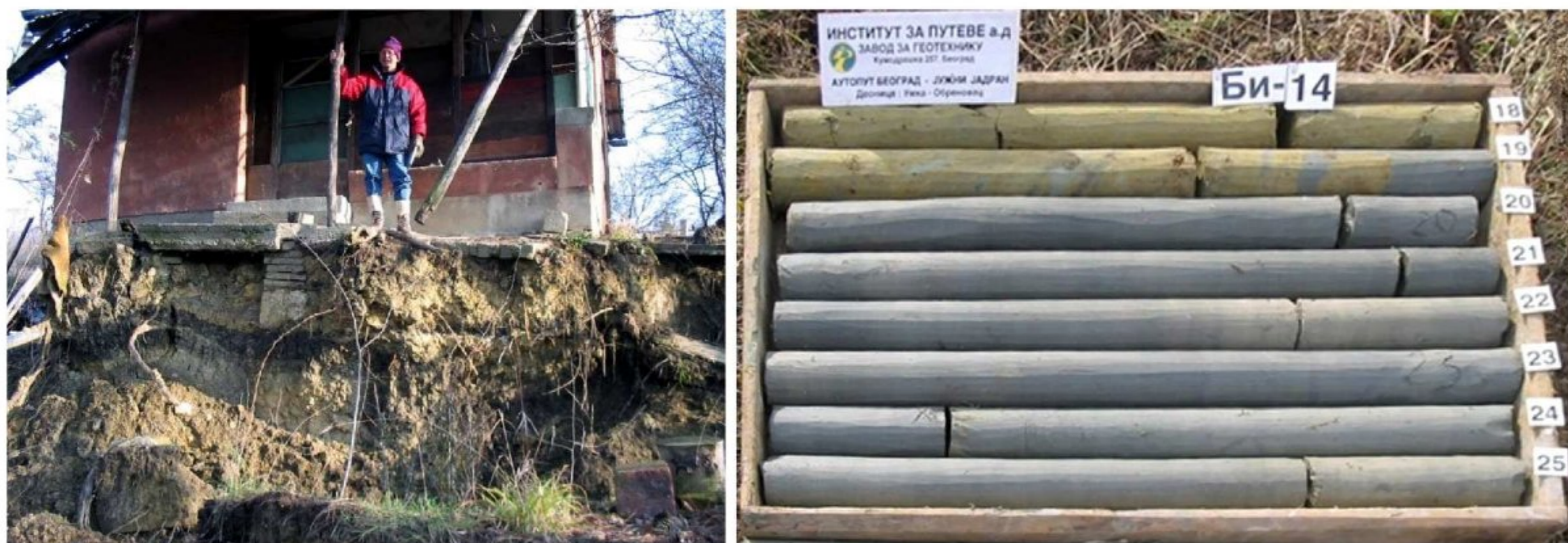
Figure 1. Field images of outcrops on the face of a secondary landslide scar, with typical remolded material with heterogeneous lenses and undulating interfaces (left); and the core box of borehole Bi 14, where interface of fresh marl and remolded clay marl, representing the slip surface, is visible (right); Photo by Svetozar Milenković.
