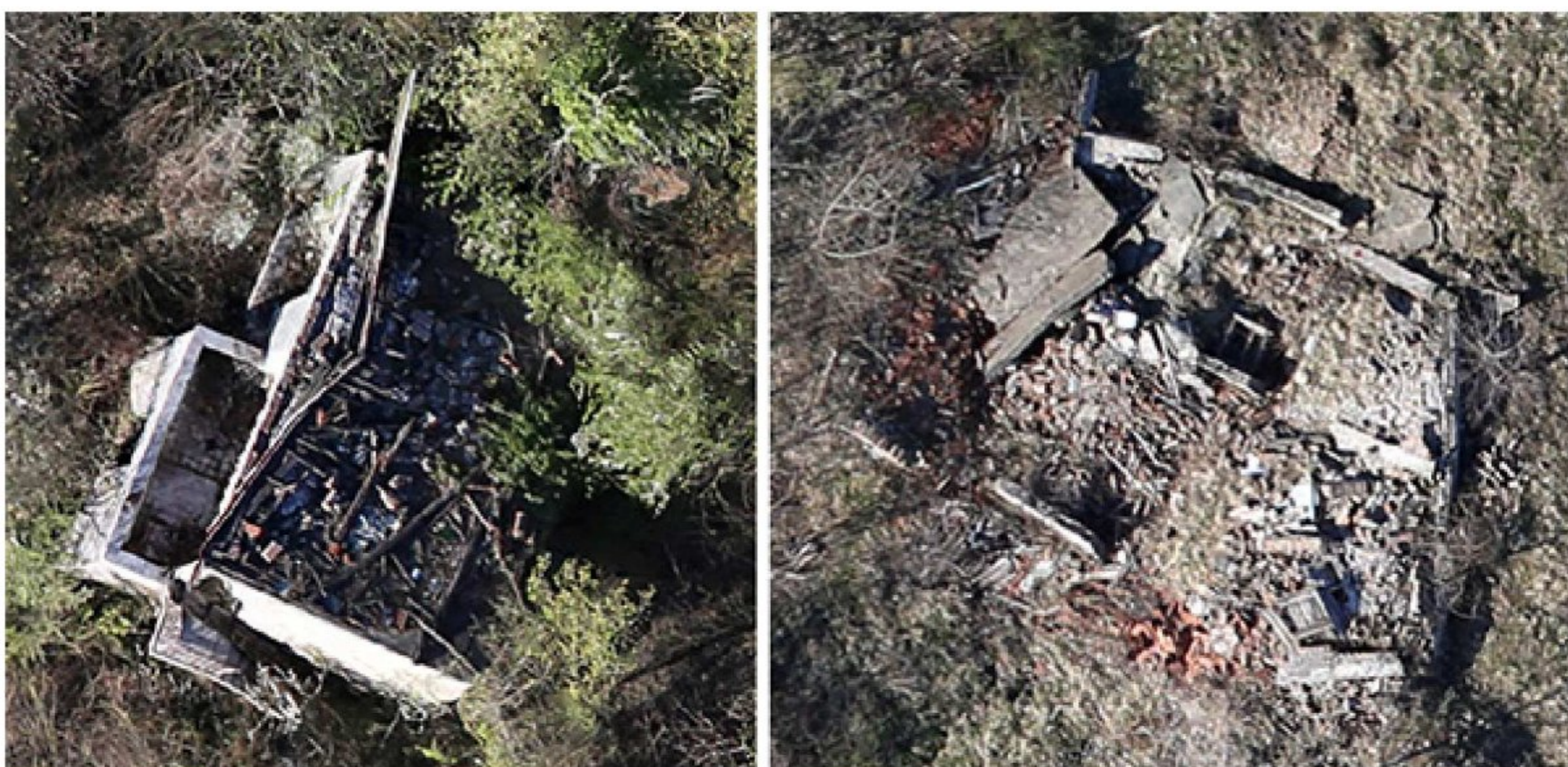
Figure 3. Aerial images of two destroyed buildings on the 'Umka' landslide that are inaccessible and surveyed by UAV remote sensing.
