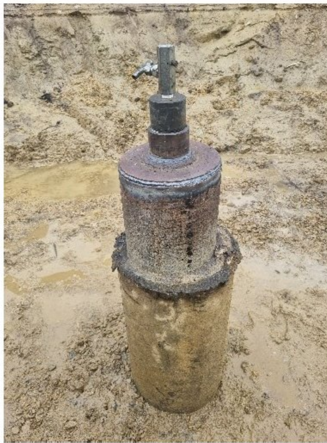
Figure 3 An abandoned well with a cover cap
