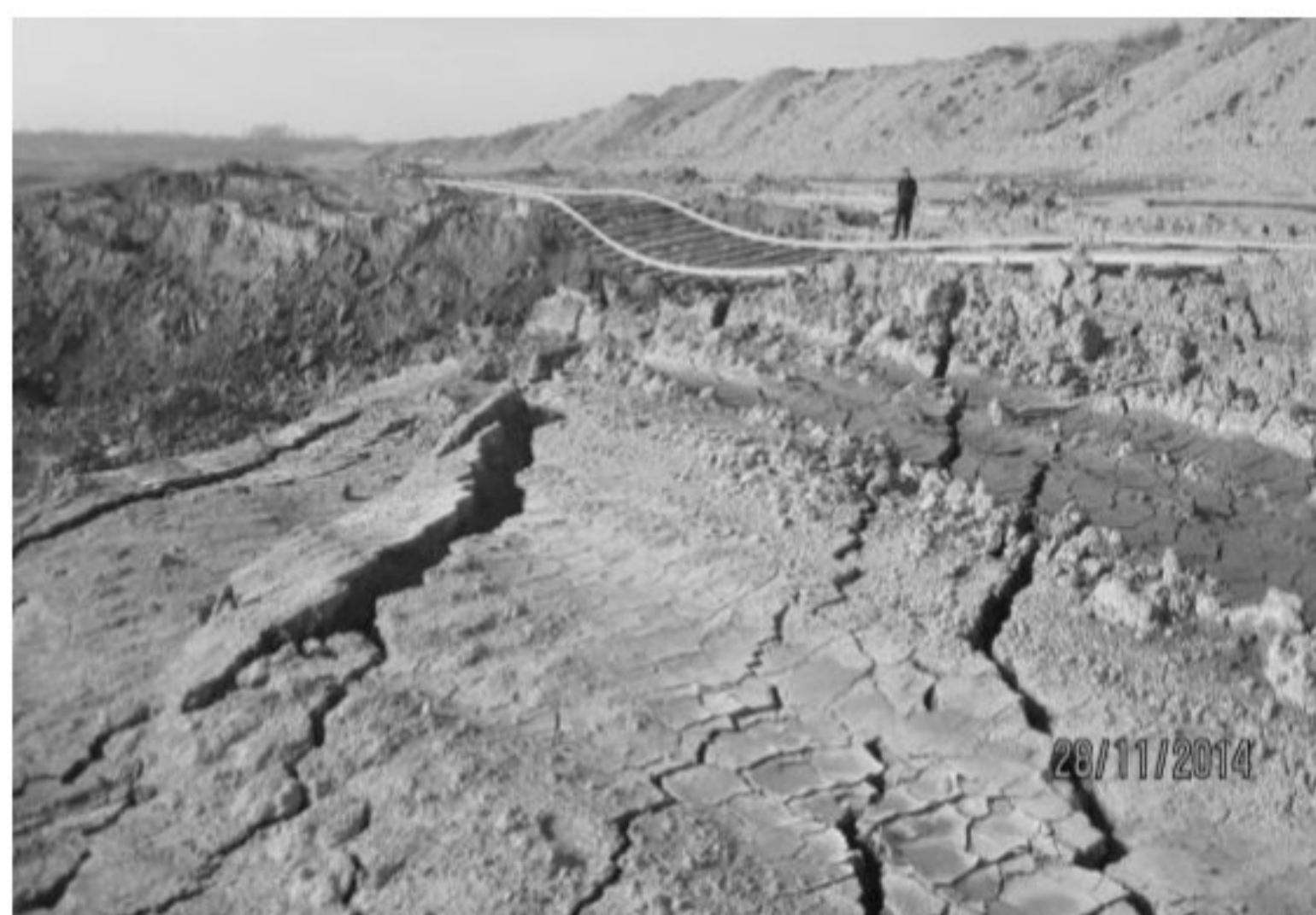
Figure 3, Damage to the O2 transporter and the route of the future Radljevo corridor
